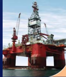
PetroRig 1 - 10,000 ft WD ( Under Construction – Singapore ) Larsen Oil & Gas
